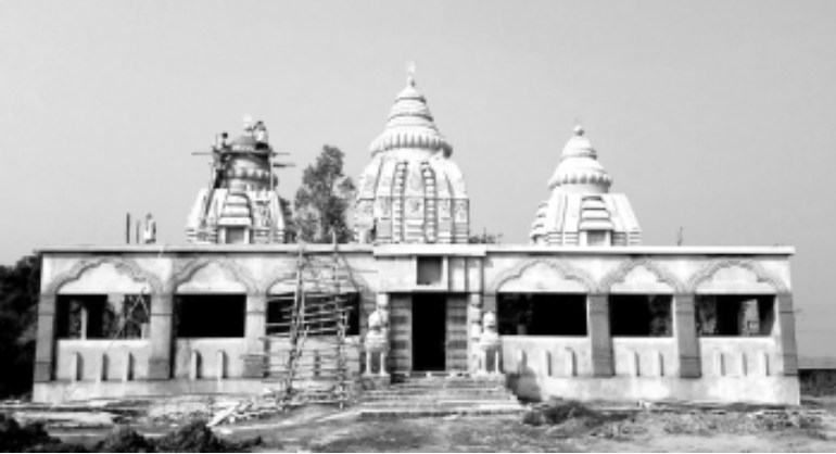
Temple Construction at Bishindipur Ashram
